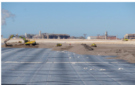
Figure 5. Sand being placed on HDPE cap
