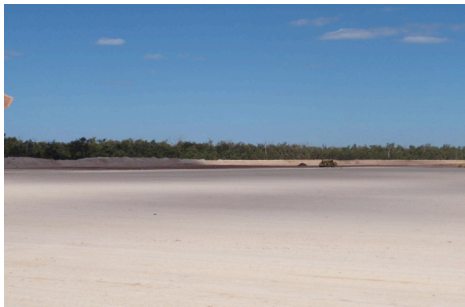
Figure 4. Clay surface prior to laying of HDPE
